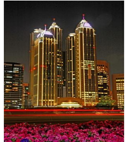
Capital Plaza Towers, Abu Dhabi Corniche
